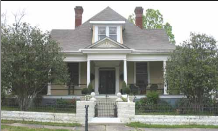
This Colonial Revival House at 304 Third Street features a full width porch with Tuscan columns and gable front projection which helps delineate the entrance area of the porch.
