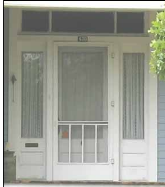
The wood screen door of this Queen Anne style house at 430 Third Street properly fits the door opening and is simple in design.
