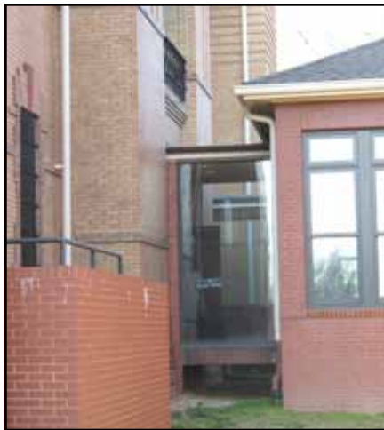
The new addition to the historic Yalobusha County Courthouse in Water Valley is illustrated the way to connect a modern addition (on the right) to the historic building (on the left) with a glass enclosed hyphen so the addition reads as separate to the historic building.
