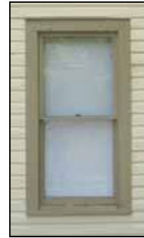
The window on the left is a classic example of a one-over-one window from a Queen Anne or Colonial Revival style house while the window on the right is an example of a two over two window also Queen Anne in style.
