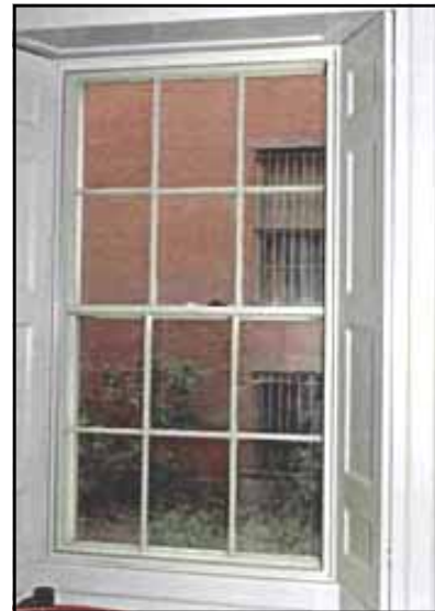
These photographs of windows in two historic houses illustrate the use of “invisible” interior storm windows. Interior storm windows are easier to remove for cleaning, are not visible on the exterior of the house, and are barely visible on the interior. Manufacturers of “invisible” interior storm windows offer storm windows that are attached either by clip or by magnetic seal, like the examples pictured above.
