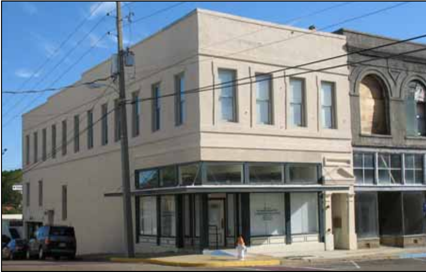
The building at 114 Main Street uses stucco on the exterior scored to look like stone blocks..
