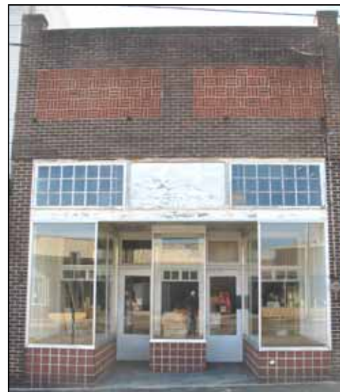
This photo of 103 Main Street shows a typical storefront from the 1920s with large plate glass windows, double recessed entry, transoms above the storefront, and wood glazed doors with transoms. These elements should be preserved to maintain the historic character of the building
