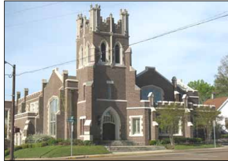
The J.J. White Memorial Presbyterian Church is a good example of the Gothic Revival style with pointed arched windows, battlements, and heavy cast stone detailing.
