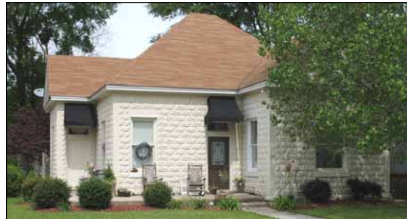
630 Virginia Avenue was constructed of decorative concrete blocks manufactured by Slader's company.
