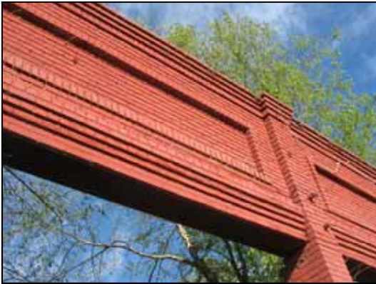
The brickwork of the parapets on several commercial buildings in McComb feature decorative brick pattering and projecting bricks to give interest to the façade.
