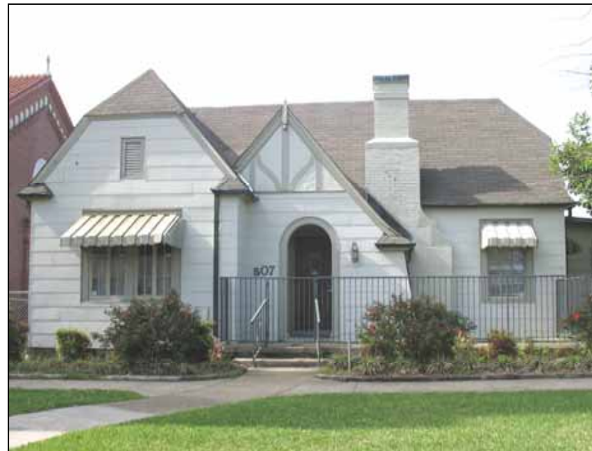
507 Delaware Avenue features a prominent front chimney and multiple high pitched gables typical of the Tudor Revival style. The front gable to the left of the door is a clipped gable.
