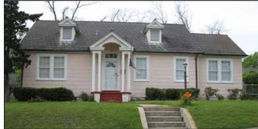
416 Third Street is a good example of the Minimal Traditional style with asymmetrical massing, low pitched roof, front facing gable roof porch, and multi-paned windows.
