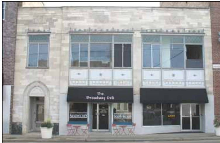
The canvas awnings on 110-112 North Broadway Street are correctly installed in the storefront opening and at the right height.
