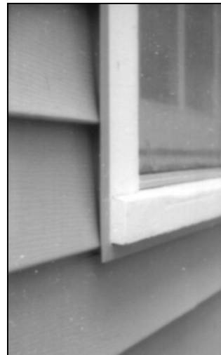
Examples of vinyl siding showing the installation of J-channels around every opening and the historic trim, if it survived the installation process.
