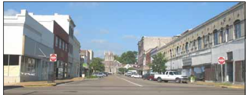
The top image (courtesy of McComb Main Street Association) shows Main Street looking west. There have been changes to the buildings over the years including the McColgan Hotel which lost its bracketed cornice when a metal slipcover was added to the building. The old Jitney Jungle has also been altered with painting of the brick, removal of a portion of the parapet, and removal of the transoms above storefront. Other historic buildings on the block have had alterations but their basic form is still intact.
