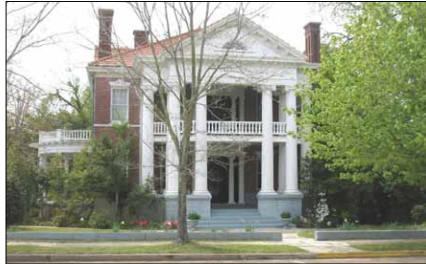
The house at 601 Delaware Avenue features a full height two-story porch typical of the Neo-Classical style.
