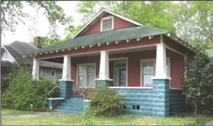
This Craftsman style house at 414 Michigan Avenue has an undercut full-width with tapered columns on masonry piers which is typical of the Craftsman style.
