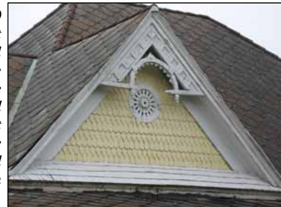
329 South Broadway Street is an excellent example of the Queen Anne style as it retains many original features including: wood double hung windows, wood lap siding, fish scale siding, turned porch columns with brackets, multi-gable roof and decorative gable brackets.
