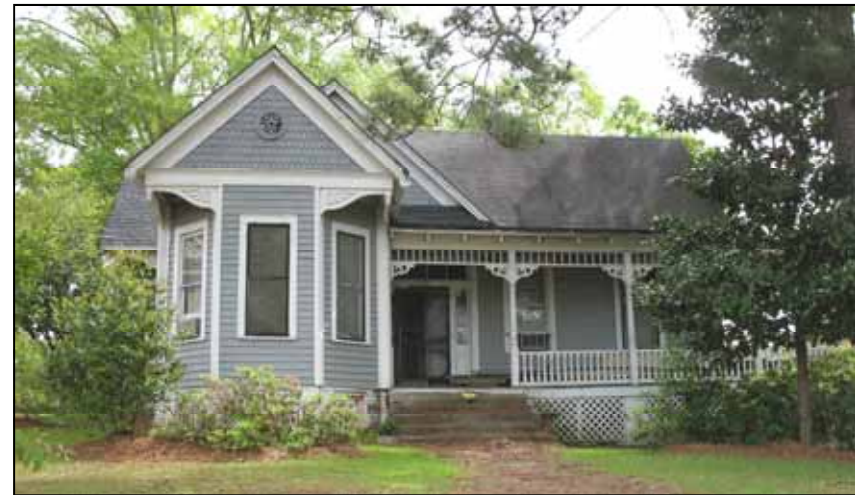
329 South Broadway Street is an excellent example of the Queen Anne style as it retains many original features including: wood double hung windows, wood lap siding, fish scale siding, turned porch columns with brackets, multi-gable roof and decorative gable brackets.
