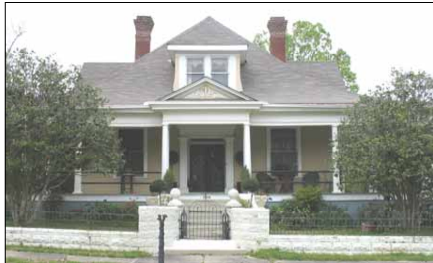
The house at 304 Sixth Street features a pyramidal roof.
