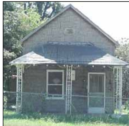
These two Natchez shotgun houses illustrate how changing the porch components alters the historic appearance and integrity of the house. The original columns on the house on the left were replaced with metal trellis columns while the house on the right has wood columns, which are also replacements but are more in keeping with original style of the building.
