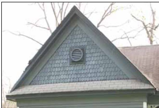
303 Magnolia Street uses a rounded shingle in the gable which is commonly known as a Fish Scale pattern.
