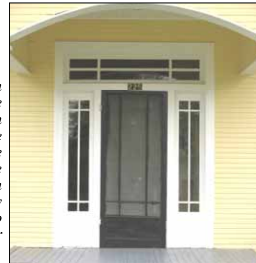
This screen door on the Craftsman style house at 225 Fifth Street is a simple design that fits the character of the house using a design pattern like the window division and it also properly fits the door opening..
