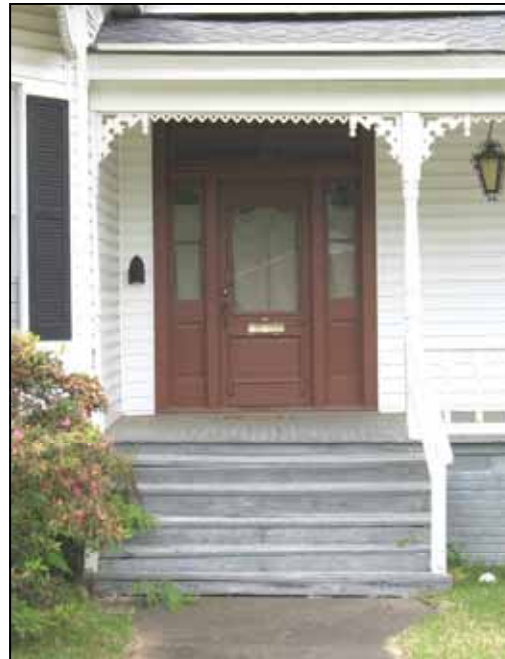
The steps of this Queen Anne style house at Fifth Street and Missouri Avenue are appropriately constructed of wood.
