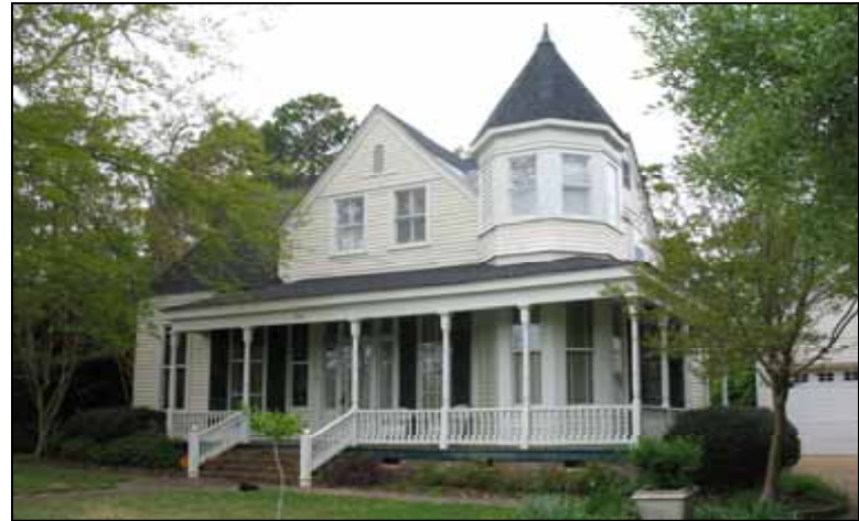
The house at 714 Third Street features a projecting wrap around porch typical of the Queen Anne style along with turned columns and a turned balustrade.
