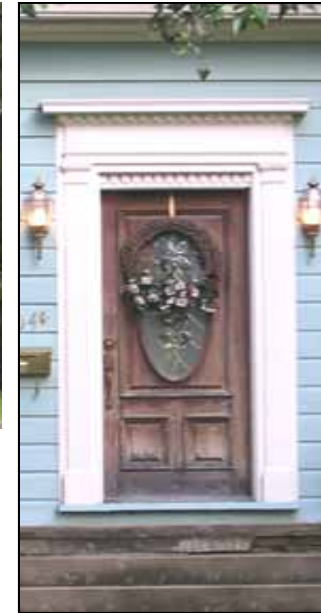
This mass-produced, leaded-glass door is not appropriate for this mid-twentieth-century Colonial Revival cottage, which would have featured a “colonial” paneled door.
