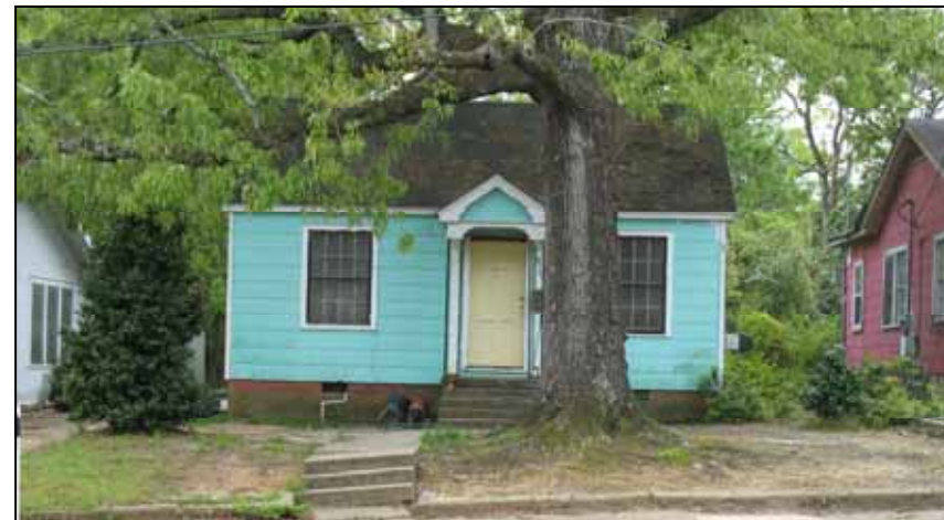
811 Missouri Avenue is smaller example of the style but still has an asymmetrical facade, low pitched roof, front facing gable roof porch, and multi-paned windows.
