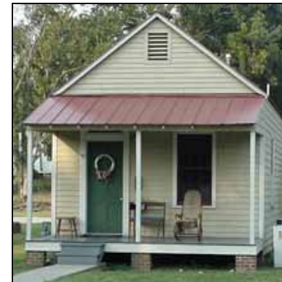
These two Natchez shotgun houses illustrate how changing the porch components alters the historic appearance and integrity of the house. The original columns on the house on the left were replaced with metal trellis columns while the house on the right has wood columns, which are also replacements but are more in keeping with original style of the building.
