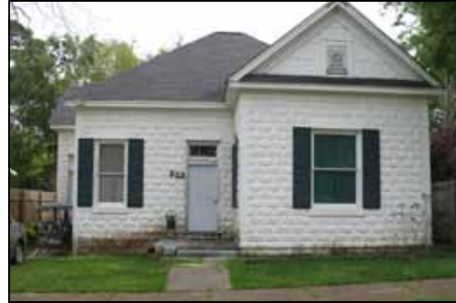
323 Sixth Street was constructed of rusticated concrete blocks which were fabricated in McComb by the B.V. Slader company. .
