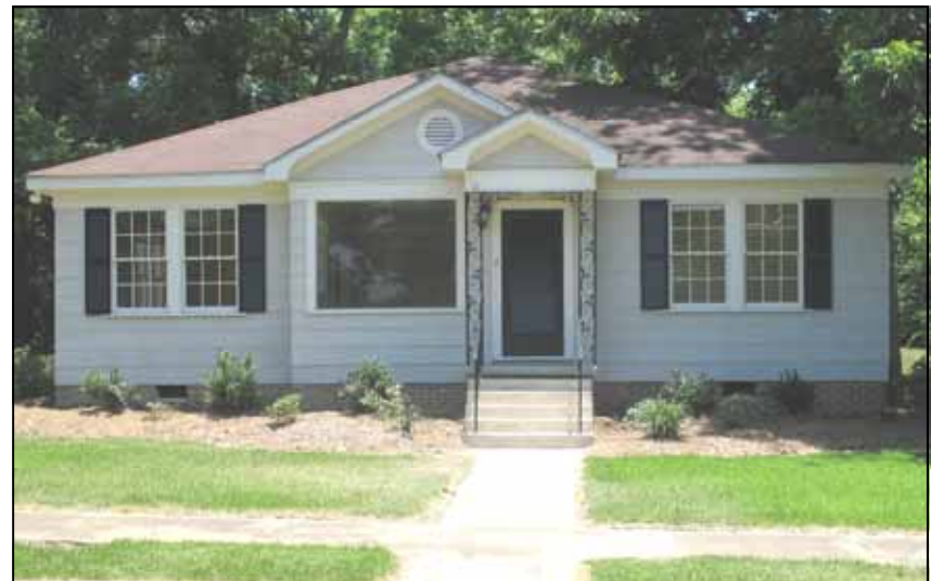
Although these applied shutters are not operable they are appropriate for this house at 515 New York Avenue as they are characteristic of the Minimal Traditional style of the house.
