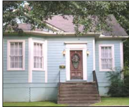
This mass-produced, leaded-glass door is not appropriate for this mid-twentieth-century Colonial Revival cottage, which would have featured a “colonial” paneled door.
