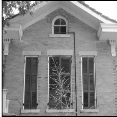
The window shutters of these two houses are original and properly fit the windows. The house on the left illustrates original shutters that are properly sized and hung for paired windows and a bay window.
