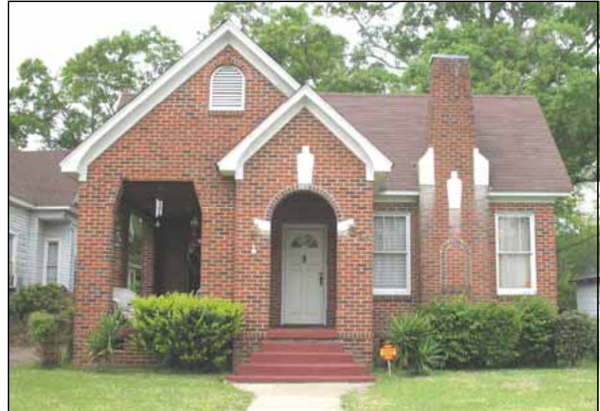
The Tudor style house at 317 North Broadway Street has two porches, a small gabled entrance porch and a larger integral porch to the left of the entrance serving as an outdoor living space.
