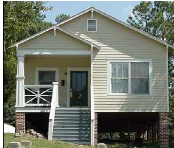
This new house built in Natchez uses Hardiplank siding to better match with the historic wood lap siding used on neighboring historic houses.
