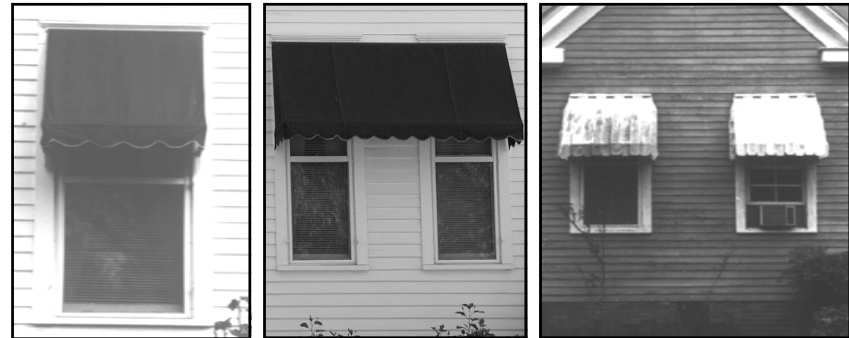
Canvas awnings are appropriate for residential buildings. The awning above left is correctly hung. The awning in the center is incorrectly hung with one awning for two windows. The metal awnings above right are incorrect for historic buildings.
