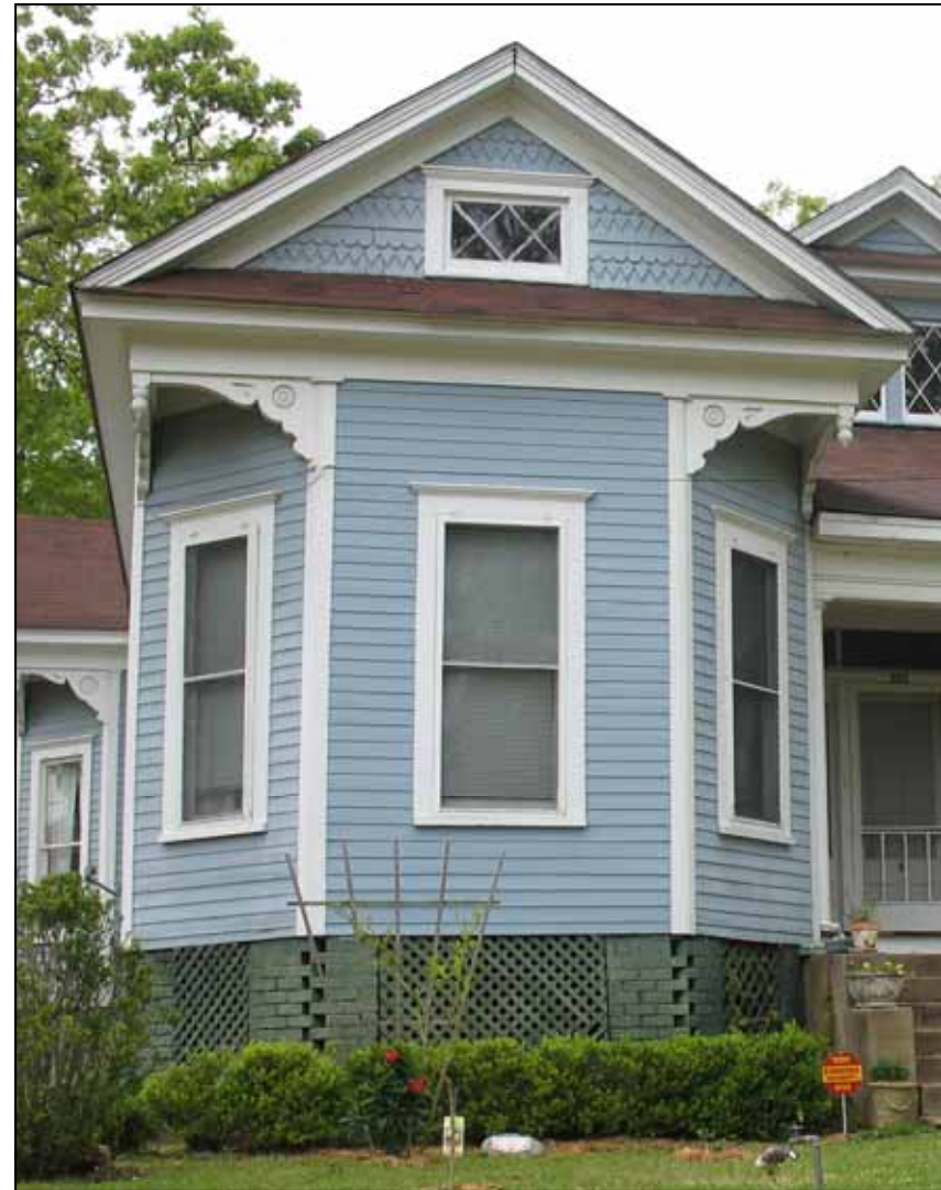
This Queen Anne style house at 430 Third Street retains its original horizontal lap siding.
