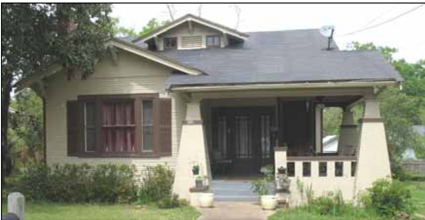
The house at 512 Louisiana Avenue is a more unusual Craftsman style house with massive tapered brick bases and small tapered wood columns supporting the porch.
