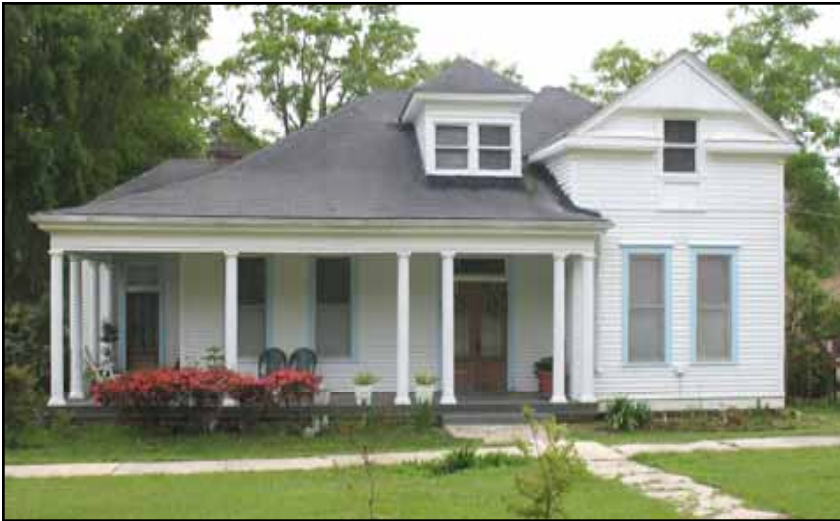
419 Virginia Avenue has a dormer with two ganged windows and a hip roof to match the pitch of the main hip roof.
