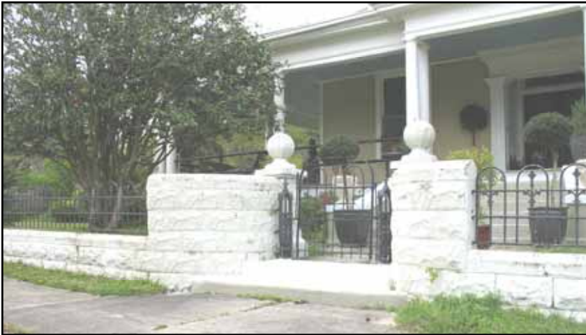
The house at 304 Sixth Street has a low masonry block wall with iron work above the wall.
