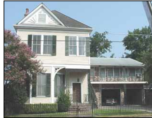
This side addition is inappropriate in proportion and scale, height, materials, massing, and roof shape. The upper and lower porches, the entrance door, and the second-story windows of this historic house have also been remodeled.
